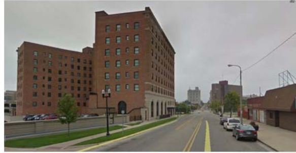
Durant Apartments – 4 blocks east and south of site
